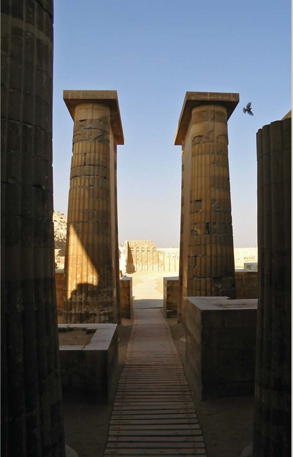
The stone columns at the entrance to the Step Pyramid were carved to resemble bundles of papyri tied together.
