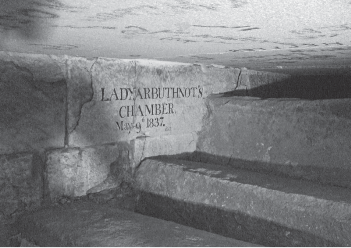
One of the relieving chambers above the King's Chamber.
