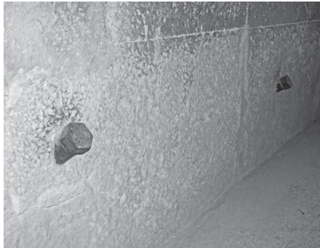
An unusual pattern of stacked blocks led to the 1986 discovery of a previously unknown chamber. The metal screw heads are stoppers for the drill holes.
