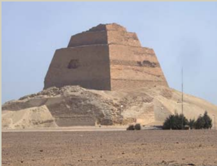
The pyramid of Meidum looks more like a fortress than a pyramid because in the Middle Ages its stones were quarried for other buildings.
