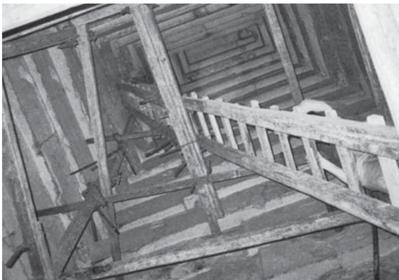
The corbelling inside the Bent Pyramid soars upward for fifty-five feet on all four sides. In the center is the ladder built by the Antiquities Service.
