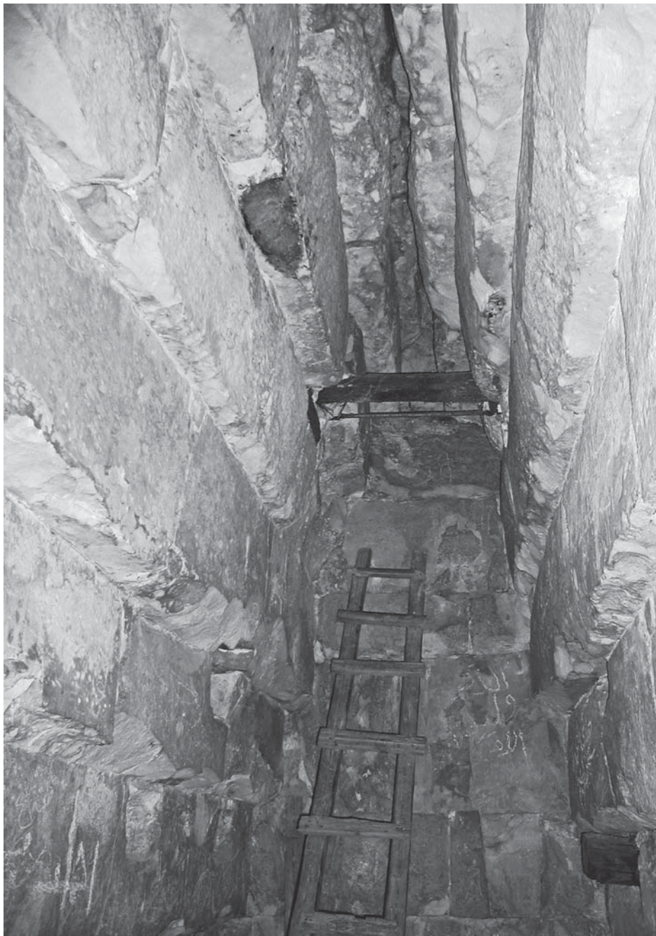
A corbelled ceiling in the Meidum Pyramid made it possible to have a burial chamber inside the pyramid.
