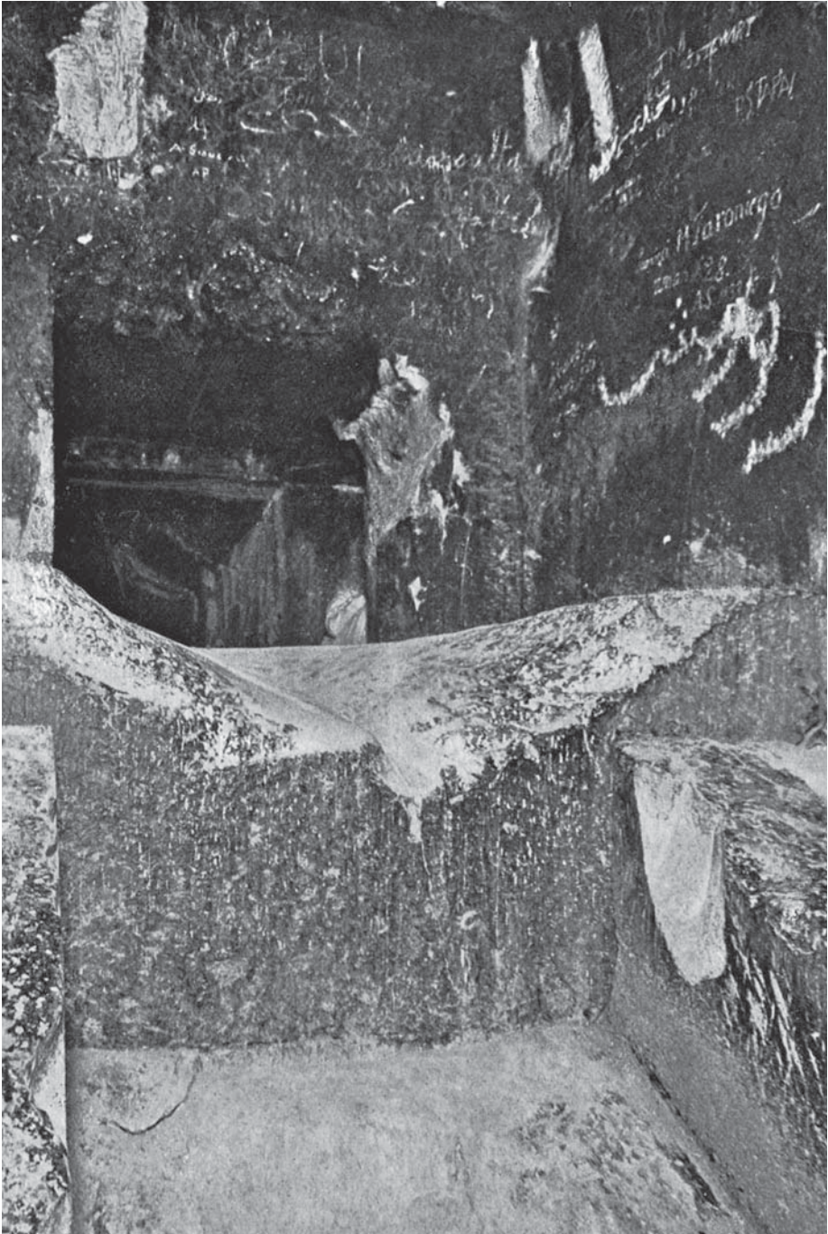
A 1911 photograph shows a groove for ropes in the large block at the top of the Grand Gallery.
