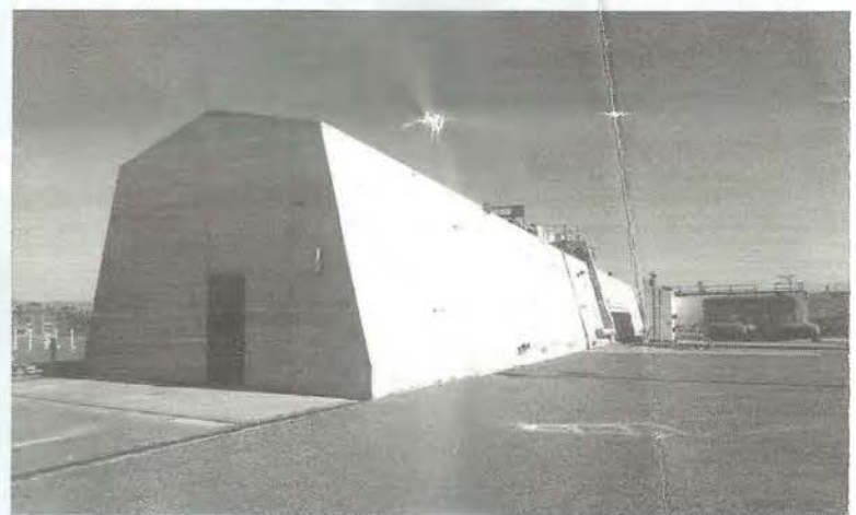
SLC-10 Launch Shelter
