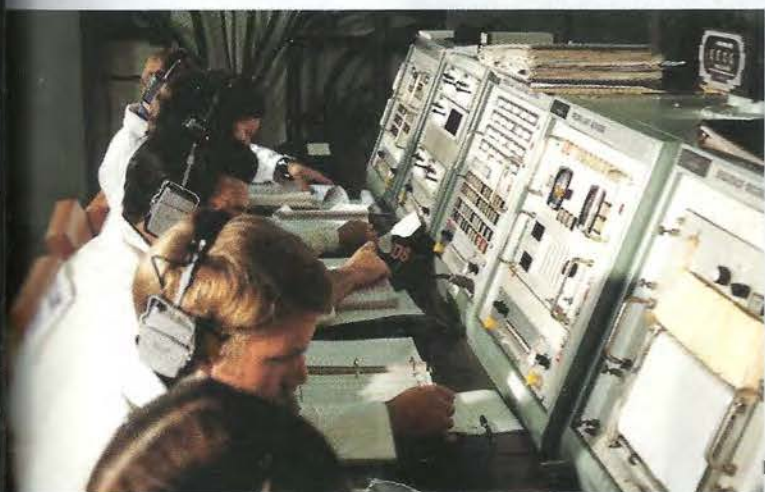
Technicians at consoles inside SLC-10 Blockhouse
